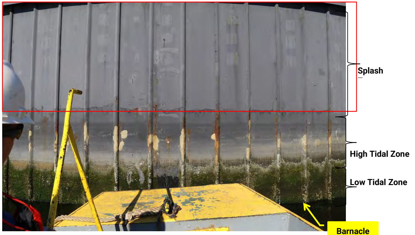
Figure 2: Photograph of Pile 13 showing mechanical damage areas in the splash zone, epoxy putty repairs at some of the corroded areas in the high tidal zone and barnacles in the low tidal zone.
