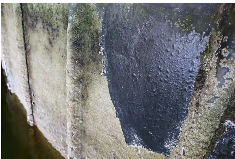
Figure 7: Photograph showing blisters in the coating after the barnacles in the low tidal zone are removed by scraping. No evidence of blisters in the coating in the high tidal zone which is free from barnacles.
