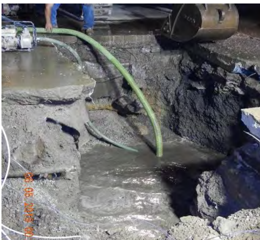
Figure 9: Photograph showing pumping out of the water to expose the 16-inch diameter pipe in the trench.
