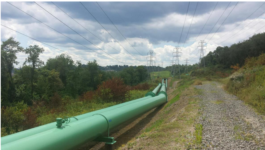
Figure 1: Photograph of aboveground natural gas pipelines co-located with electrical transmission lines.
