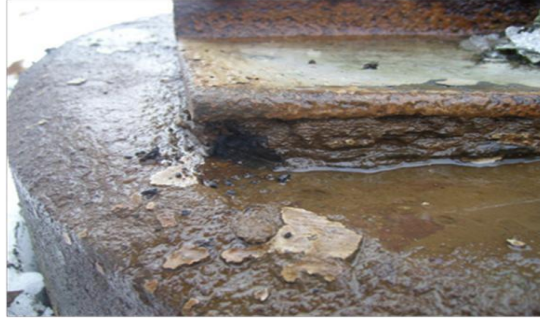
Figure 7 - Formation of pack-out between concrete foundation and base plate of WS tower.
