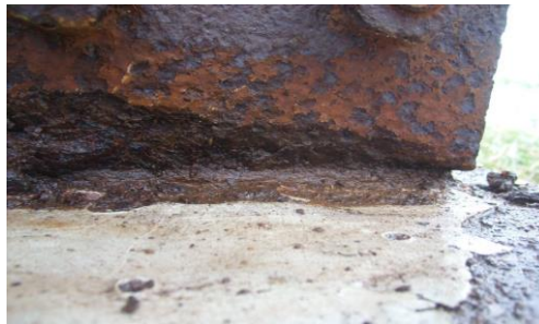
Figure 8 - Accelerated corrosion and extensive thinning of the tower leg .Was hidden under dirt/leaves
