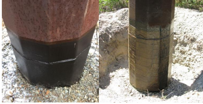
Figure 4 – Example of embedded weathering steel monopoles with field applied coating and petrolatum tape (Source: Author(s))
