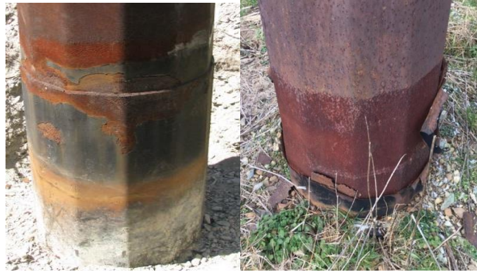
Figure 1 – Embedded first generation weathering steel poles in service for 25 years (Source: Author(s)).
