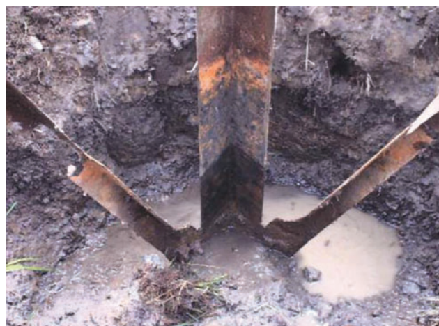
Figure 4: T&D structures located in very corrosive and water-logged soils with active bacteria present.
