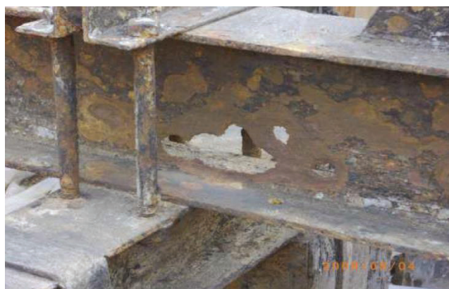
Figure 6: T&D towers in deep burial are subject to accelerated corrosion from corrosive ions.
