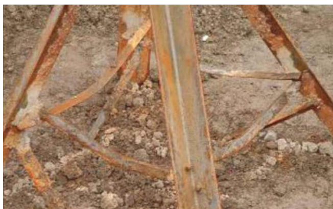
Figure 5: Corrosive backfills lead to accelerate corrosion of T&D towers.
