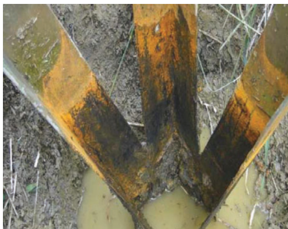
Figure 3: T&D structures may be exposed to all types of corrosion-induced environments, including MIC and stray current that require risk assessment.
