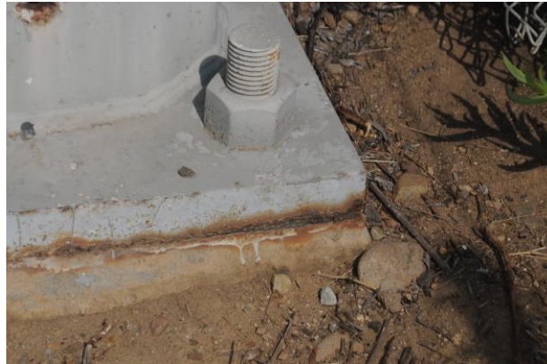
Figure 4: Photograph of galvanized based plate corroding.
