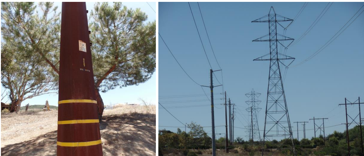
Figure 2: Weathering steel pole (left) and a galvanized steel lattice tower (right).
