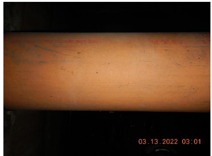
Figure 10: Photograph showing the condition of the coating on the carrier pipe.
