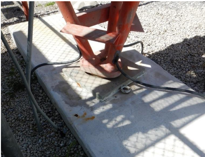
Figure 6: Photograph of the tower where the concrete foundation is open to atmosphere.
