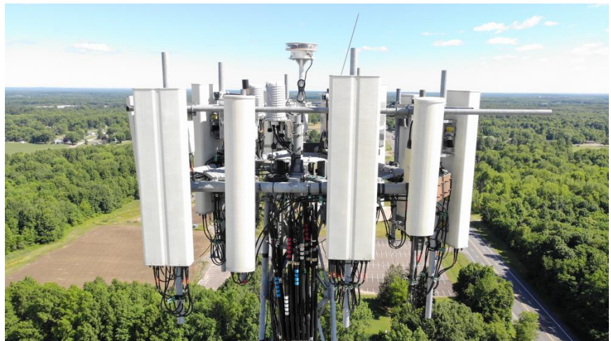
Figure 4: Photograph showing a self-standing tower and the 5G unit connected to it.
