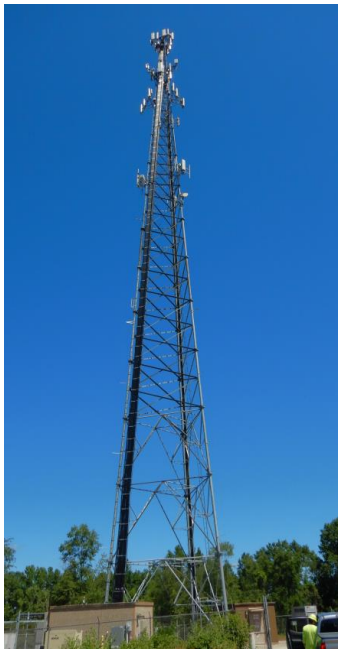
Figure 4: Photograph showing a self-standing tower and the 5G unit connected to it.
