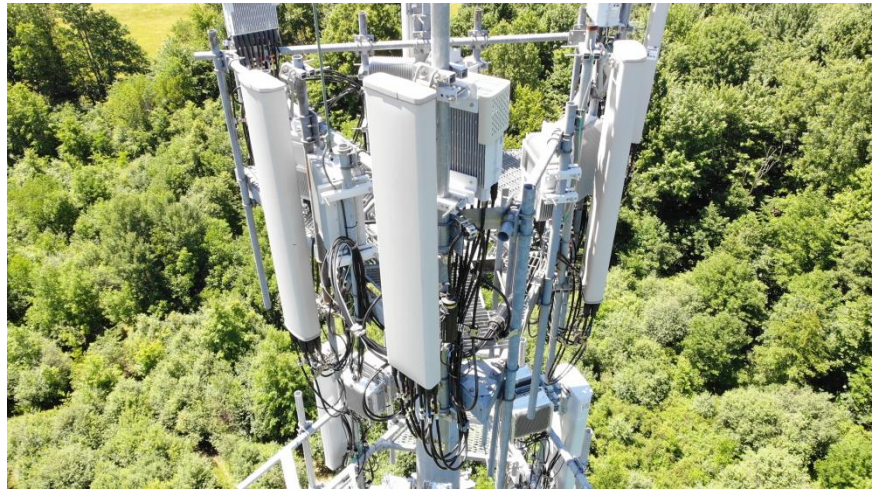
Figure 3: Photograph showing a monopole and the 5G unit connected to it.
