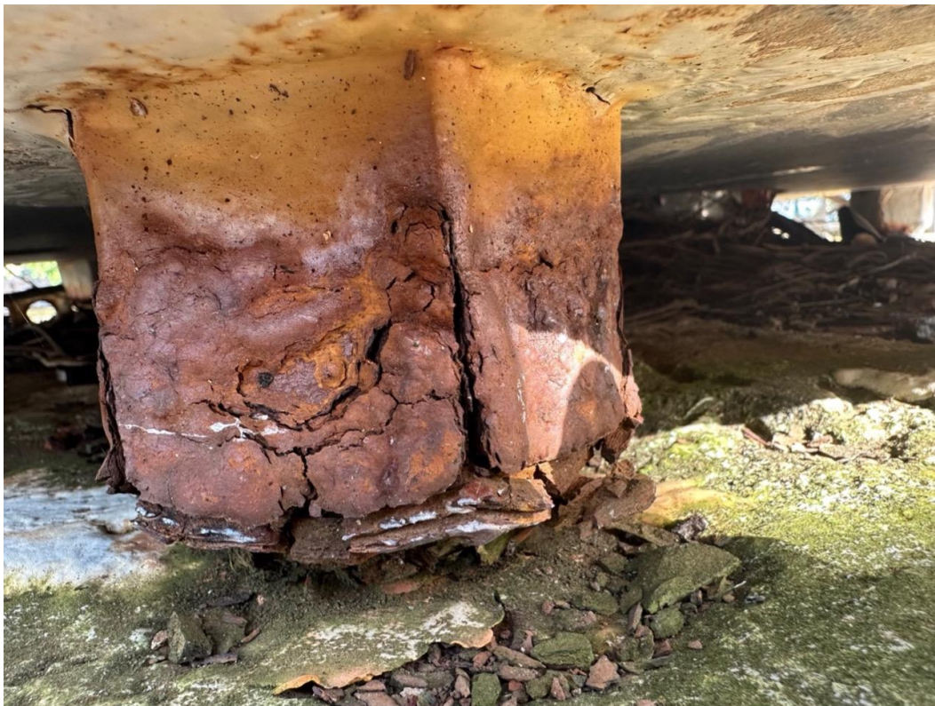
Figure 6: A galvanized anchor bolt under a base plate for a communication tower exhibiting accelerated corrosion and extensive thickness loss.
