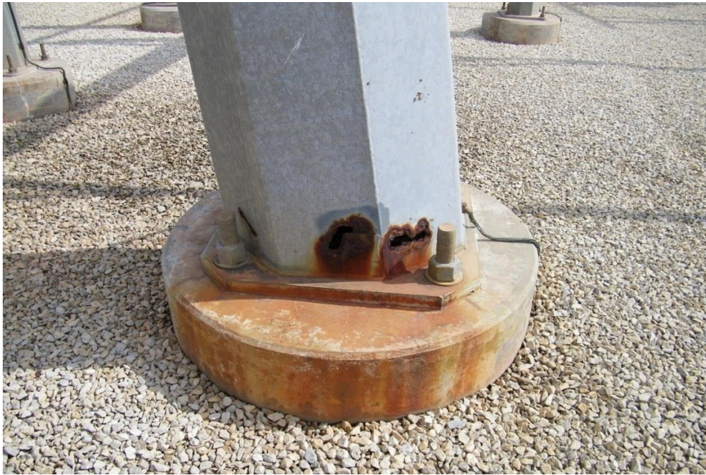
Figure 7: Internal corrosion of a substation aging galvanized pole on concrete foundation.
