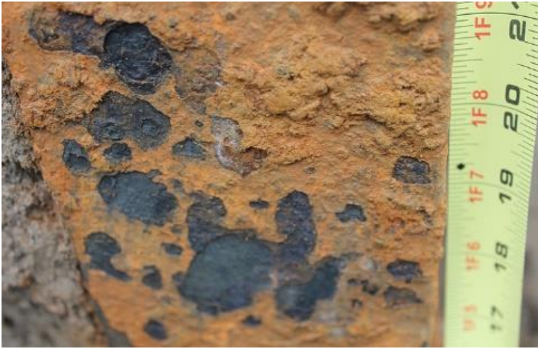
Figure 5 (b): Tower legs exhibiting signs of microbiological corrosion.
