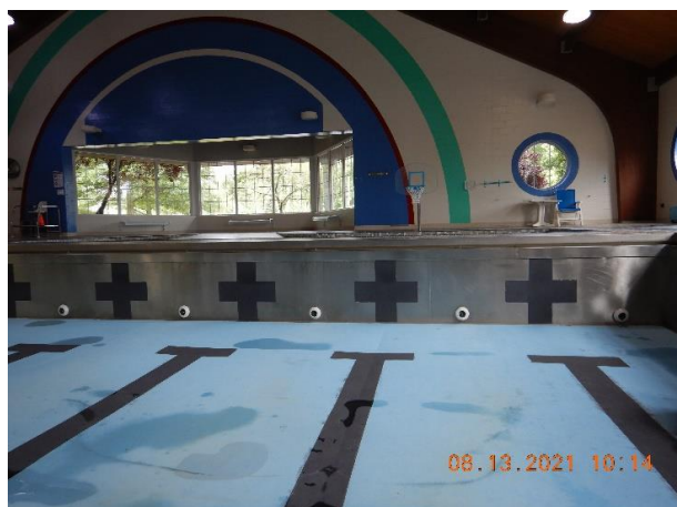
Figure 19: Photograph showing the condition of the SS material after draining the water.
