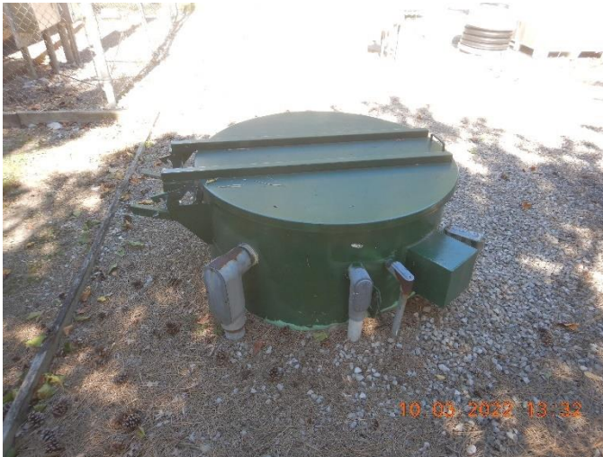
Figure 1: Photograph showing the exterior of the pump station (i.e., entrance tube) at grade level.
