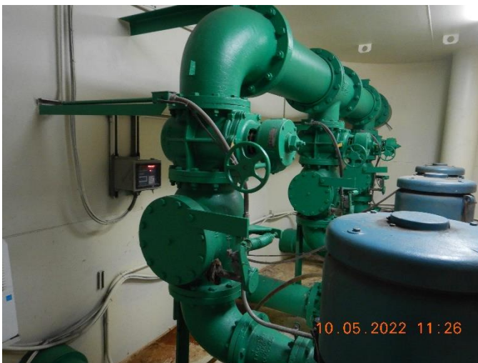
Figure 3: Photograph showing pumps and its associated piping in the pump station chamber.
