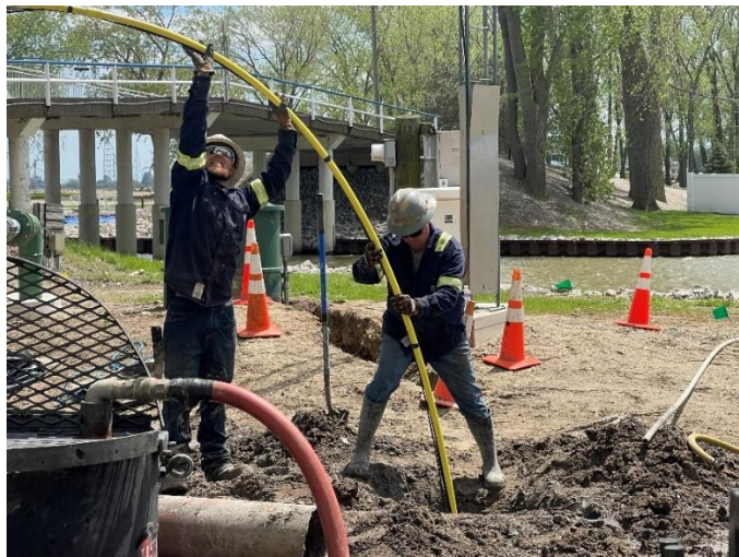
Figure 19: Photograph taken during the placement of the anodes and vent pipe in the drilled hole.
