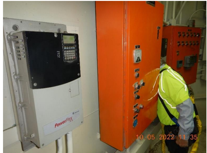
Figure 2: Photograph showing the electronic control systems essential for the automated operation of the pump station, reducing the need for direct human involvement.
