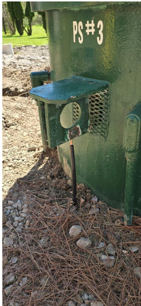
Figure 21: Photograph showing the other end of the header cable connected to the negative terminal of the rectifier is bolted to the structure at pump station 3.
