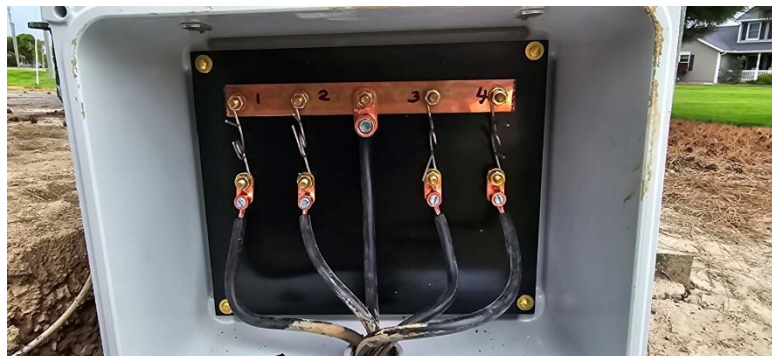
Figure 20 a): Photograph showing the junction box.
