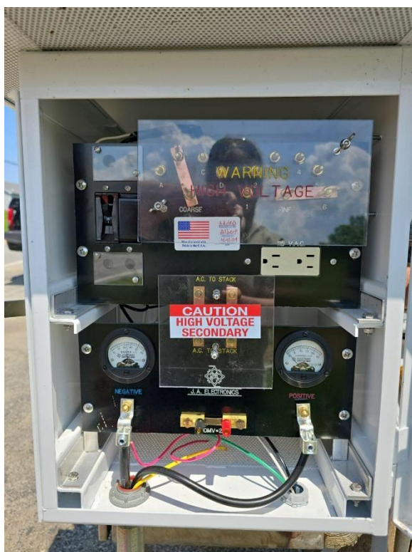
Figure 20 b): Photograph showing the rectifier.
