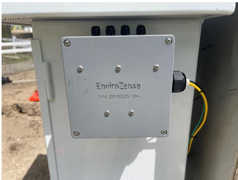
Figure 24: Photograph showing the real time structure-to-soil potentials monitoring sensor attached to the rectifier.
