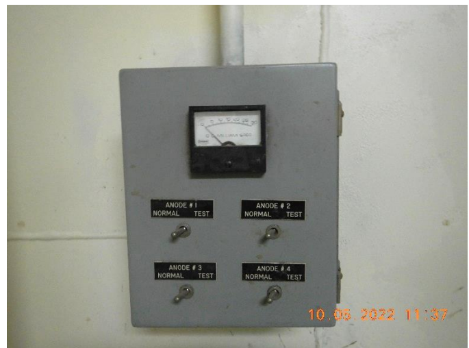
Figure 4: Photograph showing test panel for sacrificial CP system.
