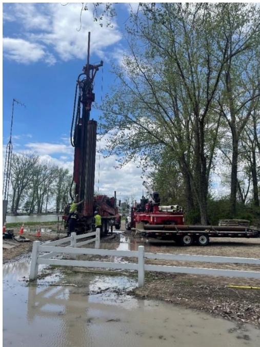
Figure 18: Photograph taken during the drilling process for anodes installation at pump station 5.
